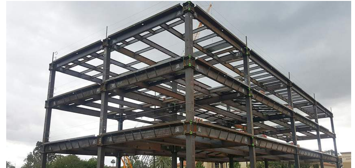
CBU ENGINEERING FACILITY STRUCTURE - CONXTECH, GENSLER
