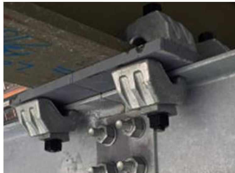
LINDAPTER CLAMPING SYSTEM AT AMERICAN COPPER BUILDING, SHOP ARCHITECTS
